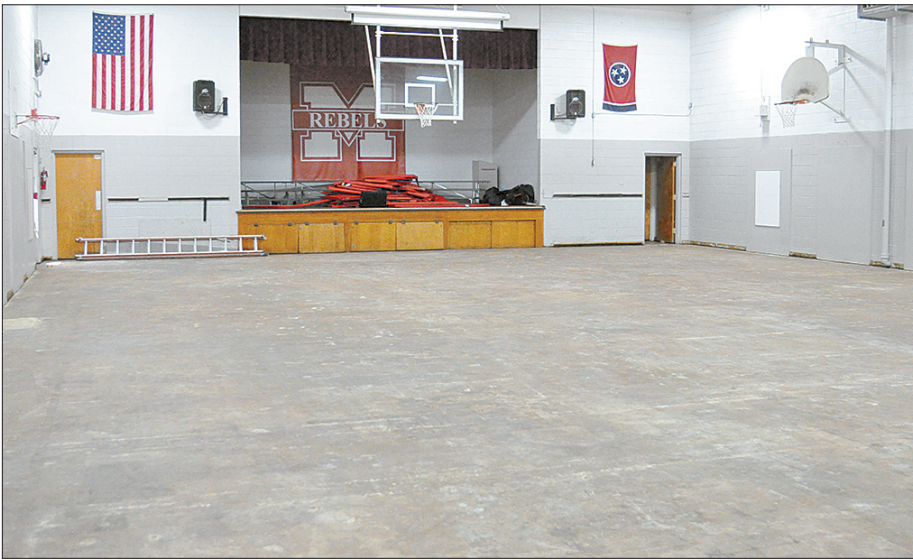
The McKenzie Elementary School gym floor has been removed and awaits the new flooring to be installed soon. Photo by Brad Sam/The Banner
