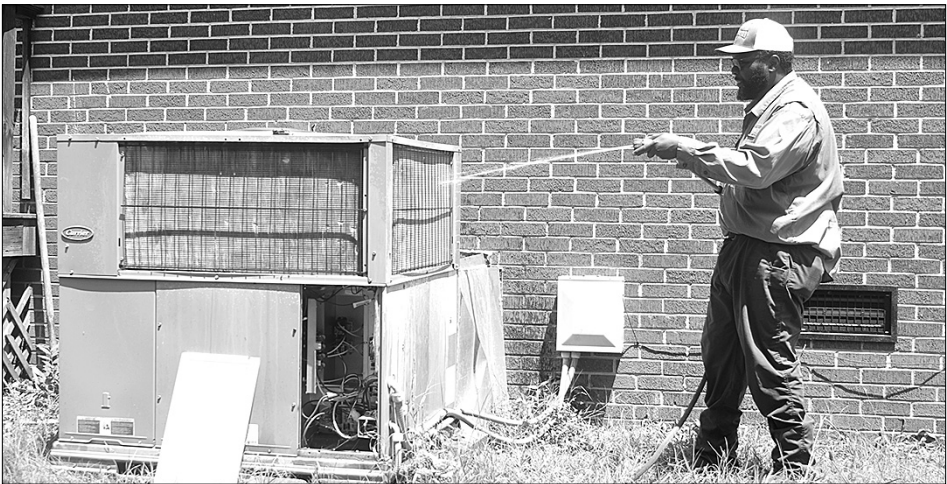
Central Refrigeration technician Michael Thomas sprays down coils as part of the maintenance of a residential HVAC unit. Photo by Brad Sam/The Banner
