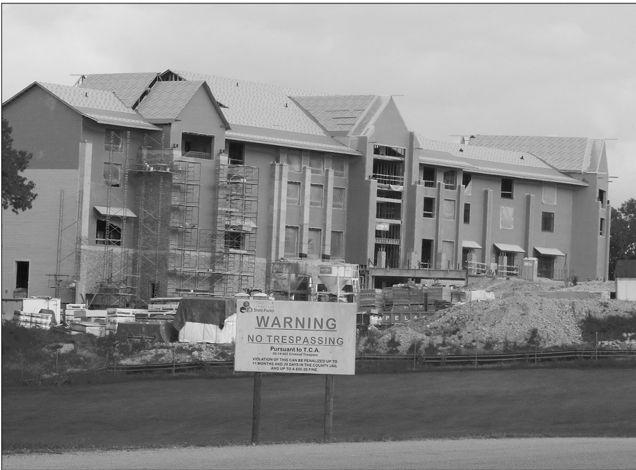
Construction of the Lodge at Paris Landing State Park continues following the park's announcement to open the lodge this fall.
