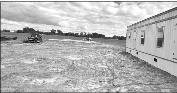
The ground clearing along with grading and the placement of housing has begun at the Hospital Wing air base located at the Carroll County Airport in McKenzie. Photo by Joel Washburn/The Banner
