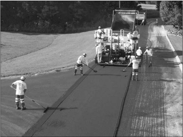
Paving was completed on Saturday at MHS by Martin Paving Company. Drone photo by Joel Washburn/The Banner
