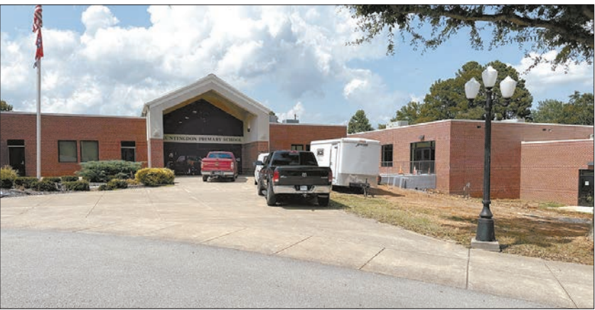
Huntingdon Primary School's addition to the building nears completion.
