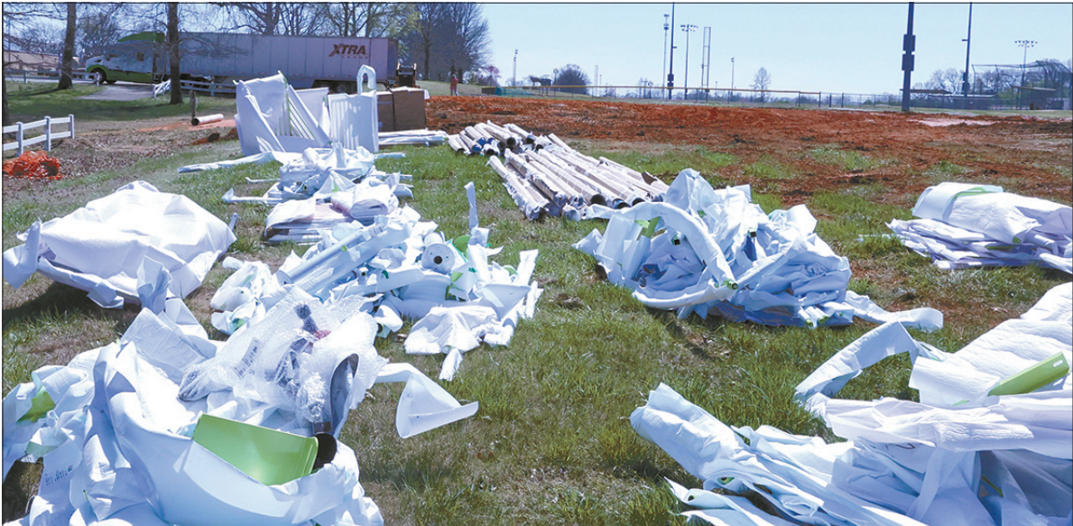
The many parts for the playground at the Carroll County Inclusion Park arrived last week on two tractor-trailers. The parts, shown here, will be assembled into various playground equipment.
