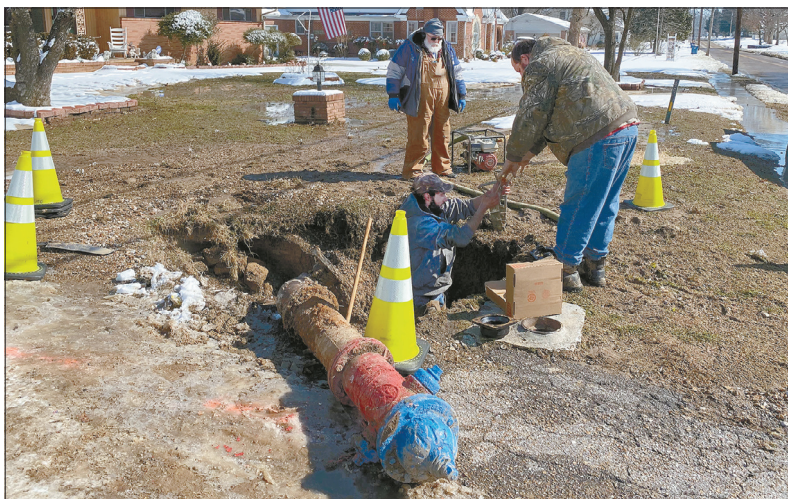
Dennis Coleman, Jr. makes repairs in the excavation, as Ernest Umstead and Billy Wood assist on ground level.
