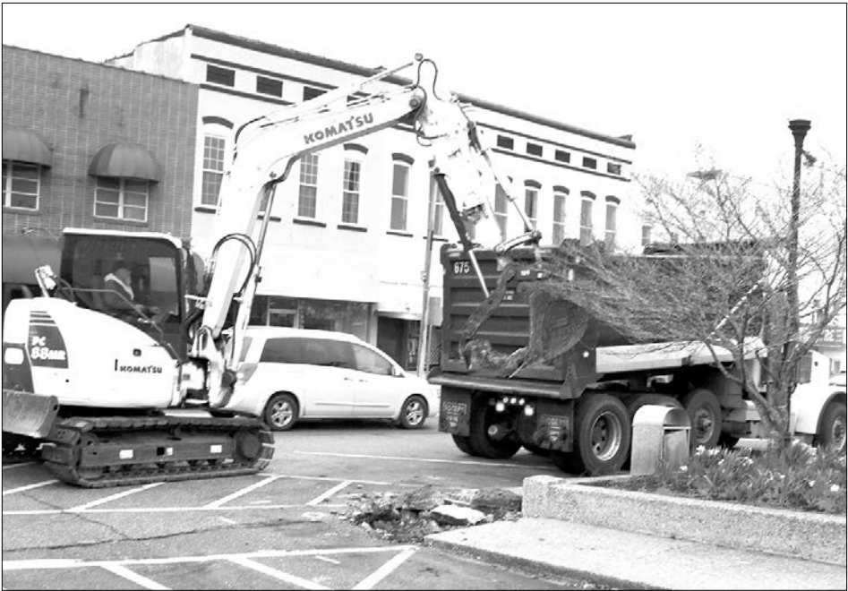
Sidewalk improvement at the intersection of Broadway and State Route 124 (Cedar) in downtown McKenzie.
