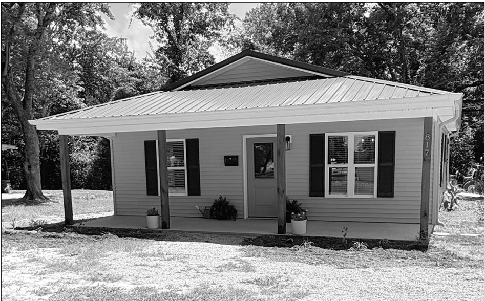
The new home of JayAnn Johnson.
