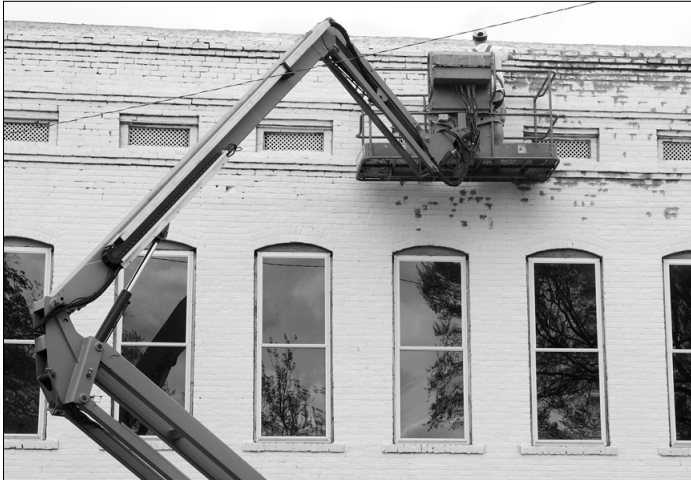
Mike Mazza uses an extendable lift to grout bricks at My Sister's Closet.
