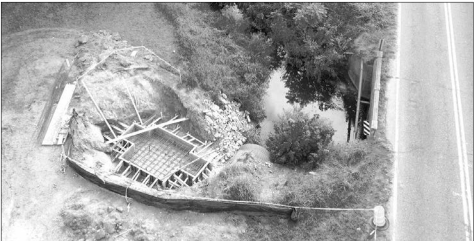
The concrete foundations are being constructed for a foot bridge over a small waterway. Drone photo by Joel Washburn/The Banner
