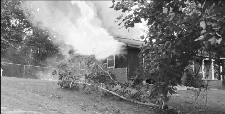
Bricks were blown from the end of the house, possibly by some type of explosion. (Photos courtesy of Huntingdon Department of Public Safety).
