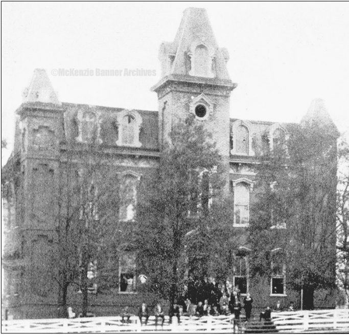
McTyiere Institute located on McTyiere St. was McKenzie's first educational institution, coming to McKenzie from Caledonia in 1867 before there was a public school and before Bethel College moved from McMoresville in 1872. It was fully accredited by the Southern Association of Secondary Schools. Originally called Caledonia College and then McKenzie College, the name was officially changed to McTyiere Institute on April 10, 1882. File photo originally published in "A Pictorial History of McKenzie, Tennessee," by The McKenzie Banner in October 2004.
