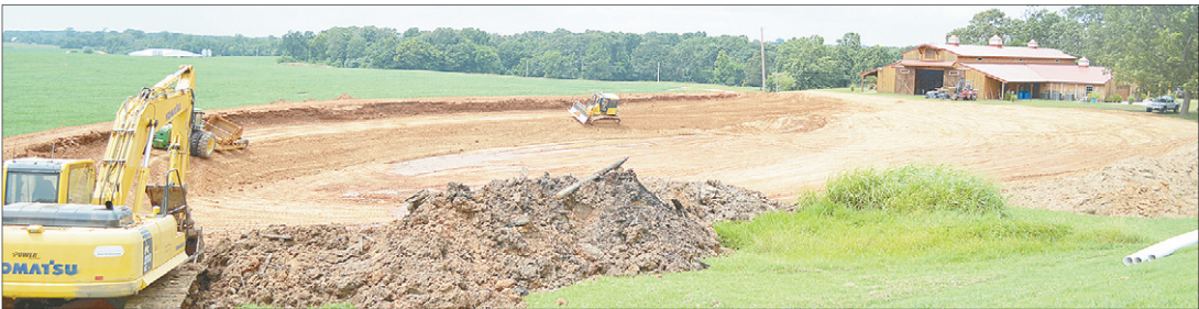
Workers from Anderson's Construction shape the pond that will enhance The Venue at Waddell Place. Photo by Brad Sam/The Banner
