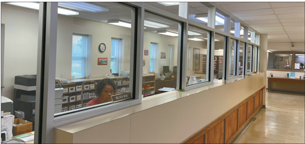
The new "germ guard" glass is installed at the Carroll County Clerk's office.
