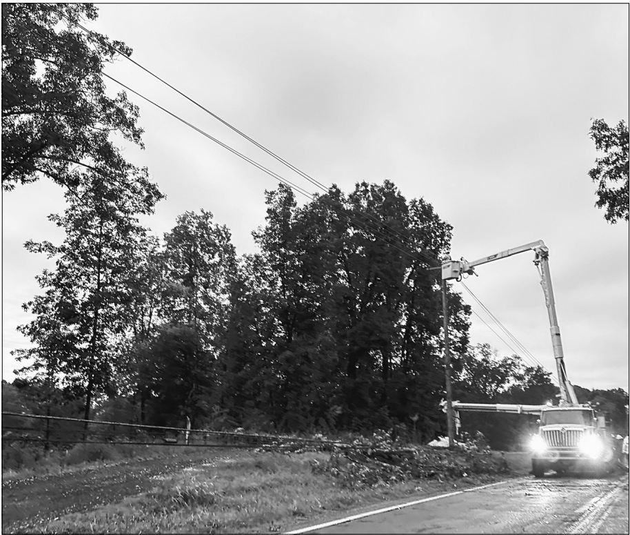
Linemen from Carroll County Electric replace a broken utility pole along U.S. 79 in Trezevant. High winds downed trees along the highway, breaking utility poles.
