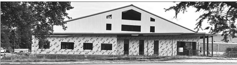
Top, All-purpose sports indoor practice facility at McKenzie High School. Above, Christian Family Medicine and Pediatrics new building on Highland Drive. Below, Bethel University's new 1,058 seat chapel.
