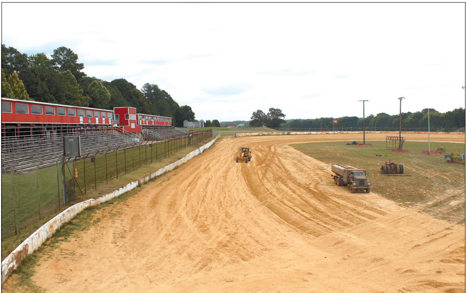
The Clayhill Motorsports Park team is working diligently to repair the 3/8 mile racetrack in Atwood before the July 27 Test and Tune.
