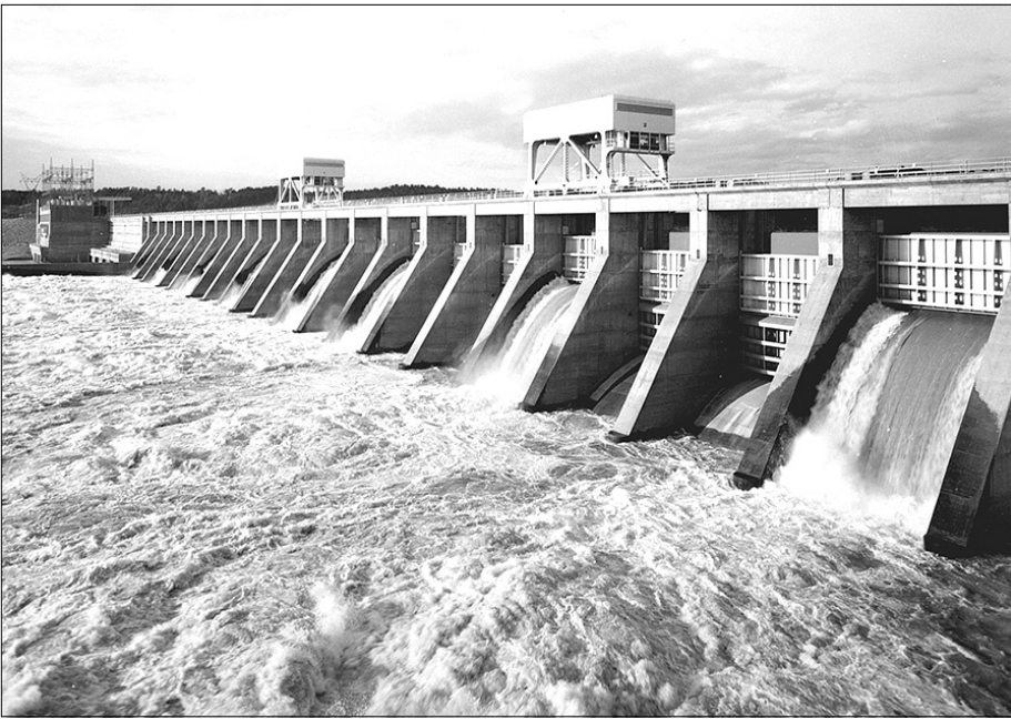
Pickwick Landing Dam is a hydroelectric dam on the Tennessee River in Hardin County. The dam is one of nine dams on the river owned and operated by the Tennessee Valley Authority.
