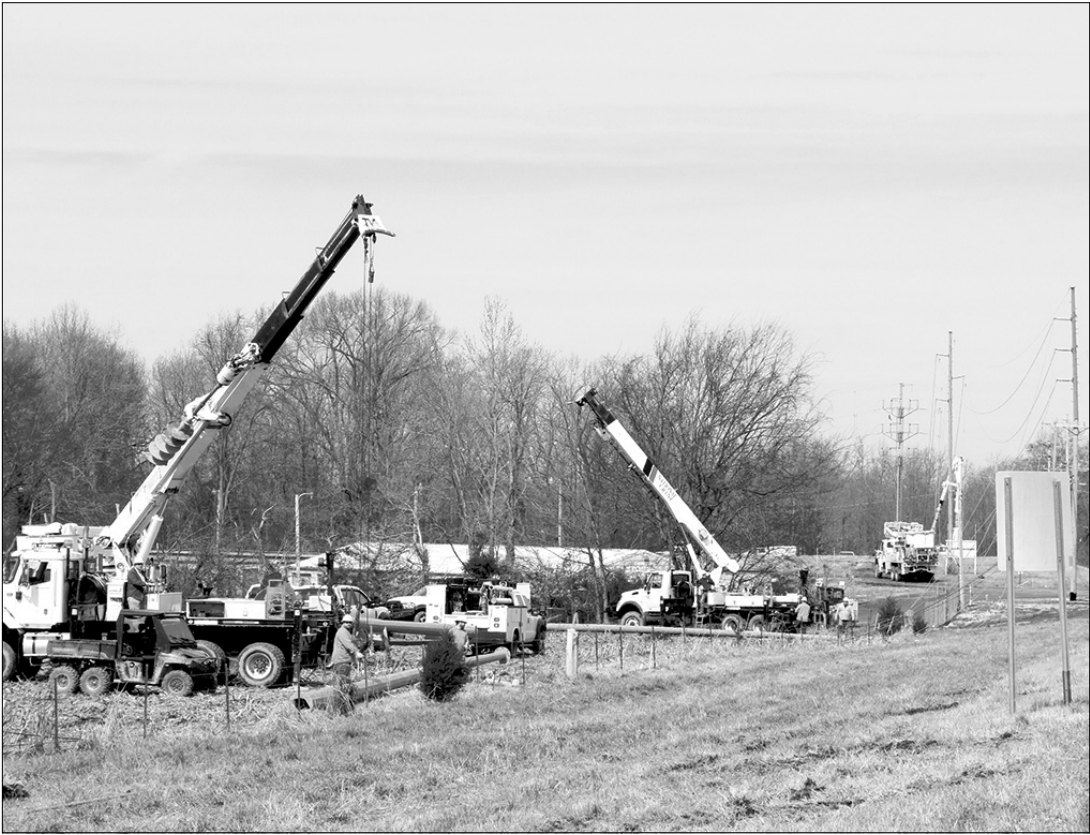
Above, The Steve Jackson home on Newton Road, McKenzie was totally destroyed. The tornado left a debris field for 100s of yards. Below, Contract crews erect new 75-foot metal power poles along State Route 22 near Carroll County Airport. The poles had 69,000-volt lines that served the substation at the airport. Carroll County Electric connected to Weakley County Municipal Electric to provide electricity to the McKenzie area until the power lines could be restored.
