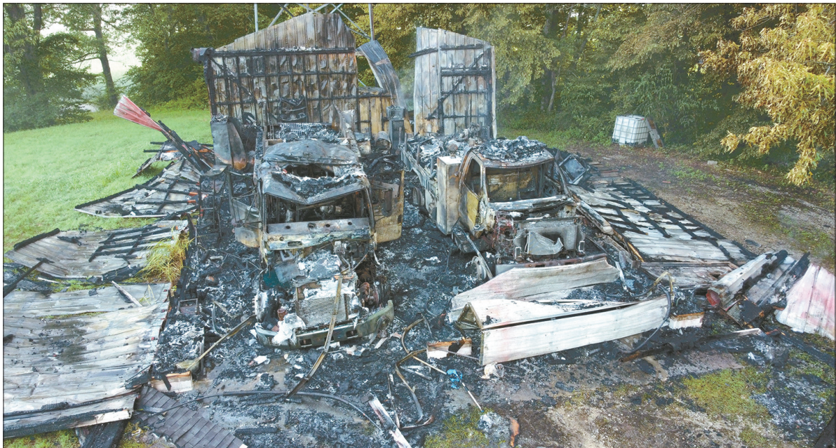
The day after the fire from an overhead drone photo. The building and two trucks are destroyed. Photo by Joel Washburn/The Banner
