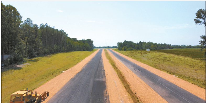
Construction on the State Route 76/U.S. 79 bypass around Atwood is progressing. This is a aerial photo of the roadway near West Carroll Junior/Senior High School in Atwood. Photo by Joel Washburn/The Banner
