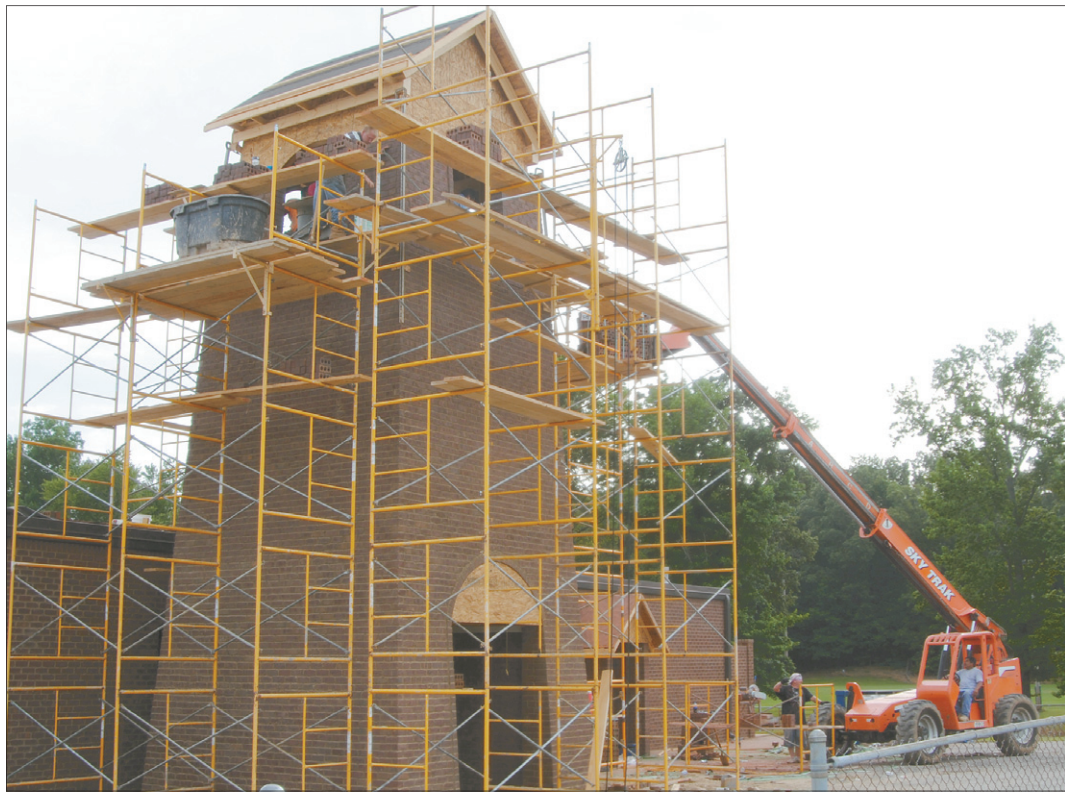
Work nears completion on the fieldhouse bell tower.
