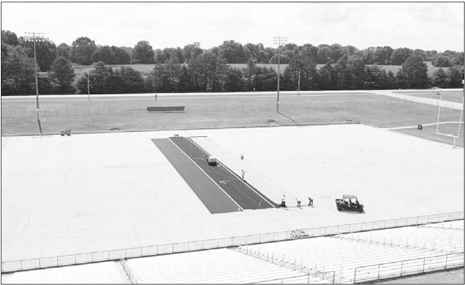
In the second week of Bethel University's turf replacement project at Walter Butler Stadium, the football field was completely stripped of its decade-old turf. The football field's turf removal process began Monday, June 15, and crews have now begun placing new turf on the field. In March 2026, Bethel University's Vice President of Athletics, Derek Horne spoke to the McKenzie Rotary Club about the project, noting that the school's primary concern is ensuring the safety of student athletes. Officials told The Banner that the new turf must be placed by July 15 for the return of football players for preseason activities. Drone photo by Joel Washburn/The Banner
