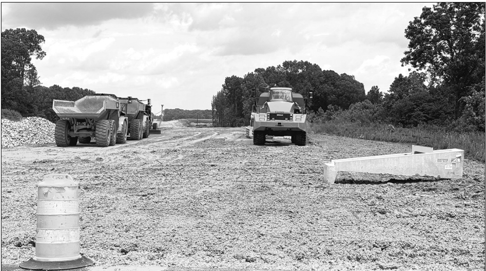
A photo of the construction work on State Route 76/US 79 as pictured from the intersection of State Route 105 in Trezevant. Photo by Joel Washburn/The Banner
