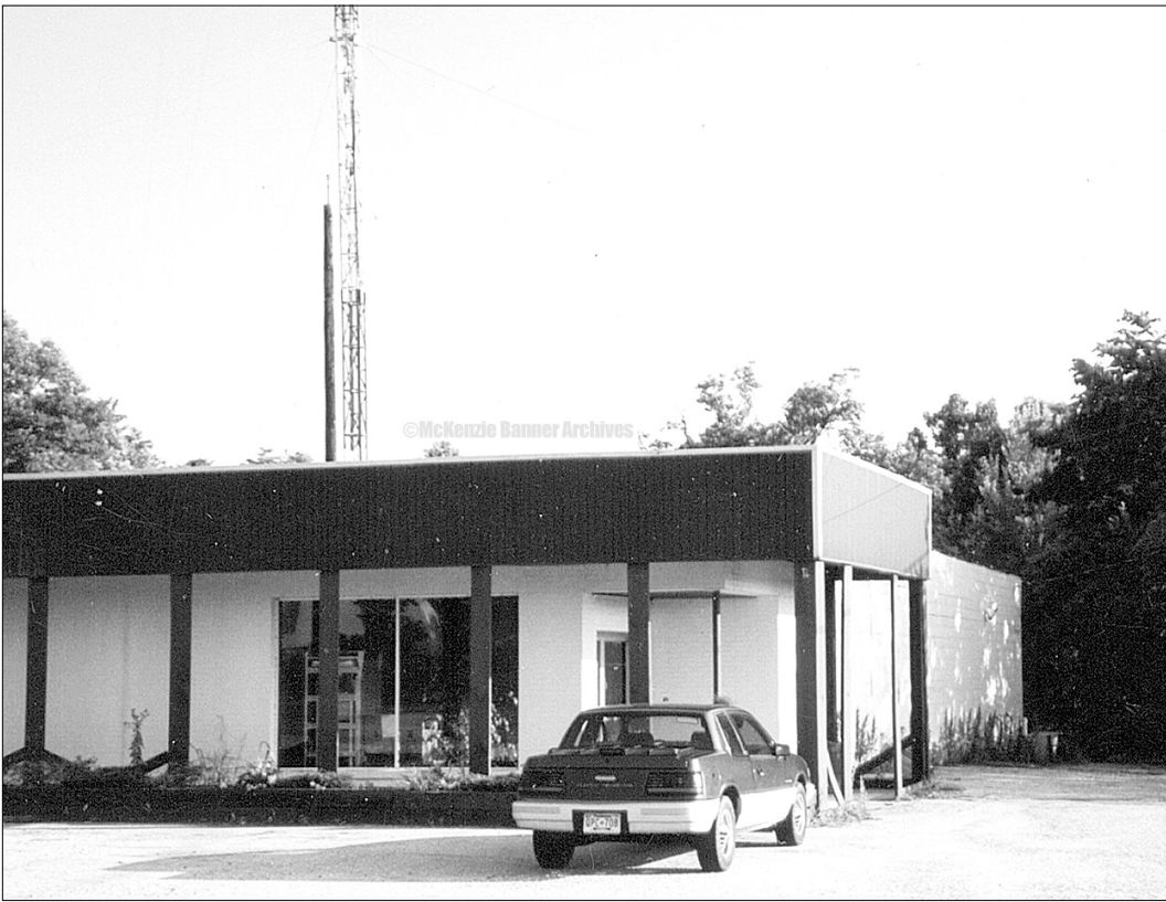
WKTA-FM Radio Station occupied the former Drewry's Food Center building in the 1980's. File photo originally published in "A Pictorial History of McKenzie, Tennessee," by The McKenzie Banner in October 2004.
