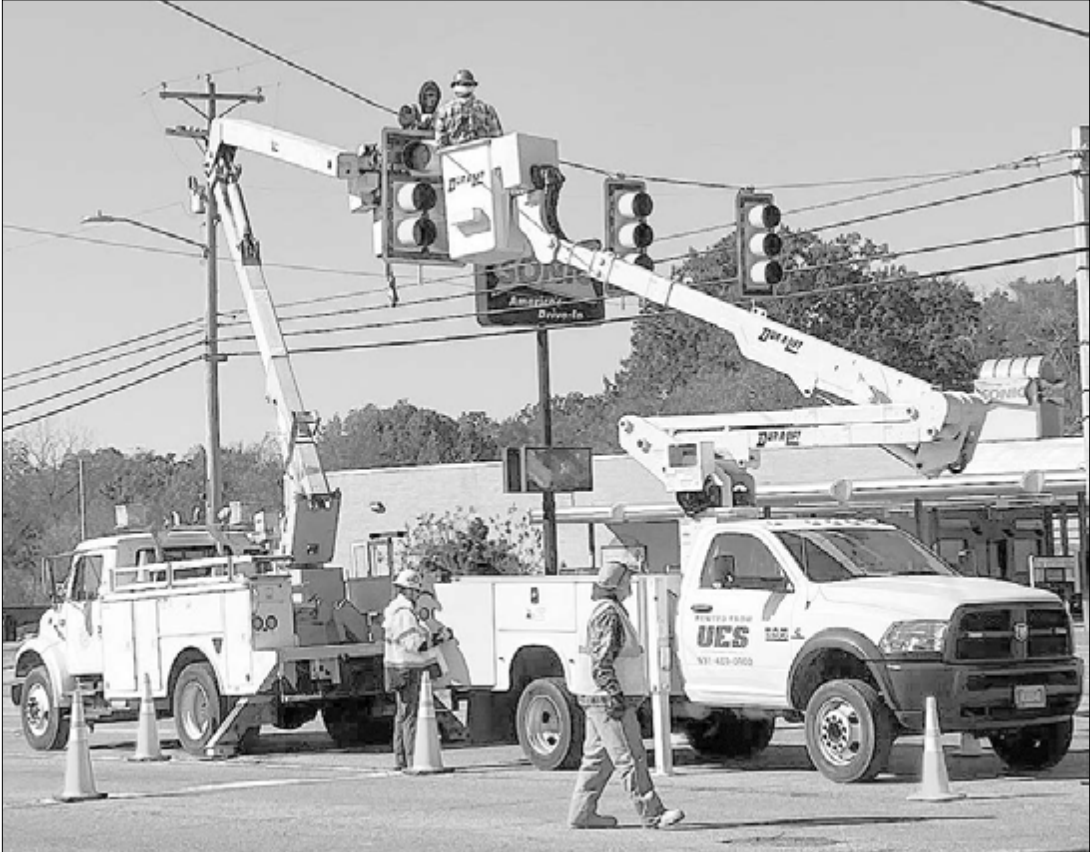
Crews subcontracted by Trane work in conjunction with the City of McKenzie to replace signal lights on Highway 79 in town.
