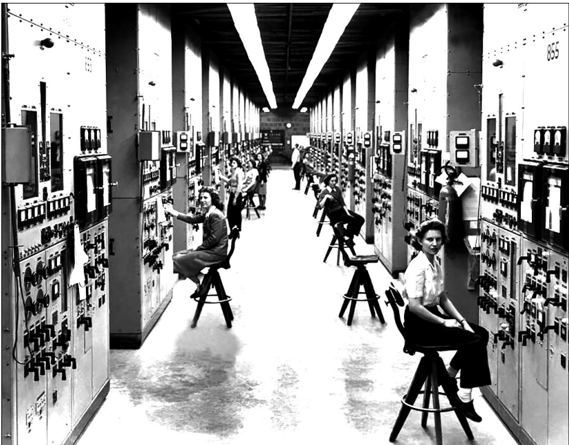
Above Left, Calutron operators sit at their panels unknowingly refining uranium ore into fissile material. Galerie Bilderwelt/Getty Images Above Right, X-10 Graphite Reactor, Oak Ridge, Tennessee. Below Right, A shift change at the Y-12 uranium enrichment facility in Oak Ridge. Galerie Bilderwelt/Getty Images
