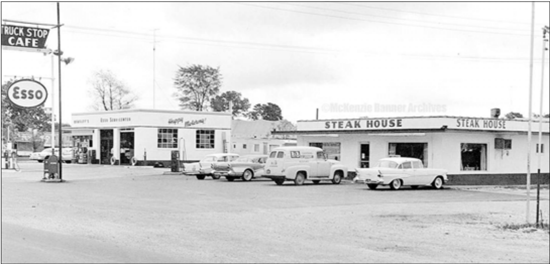
The Steak House, owned and operated by Billy Vawter, Highland Drive, late 1950s and BEASLEY’S ESSO SERVICENTER. File photo originally published in “A Pictorial History of McKenzie, Tennessee,” by The McKenzie Banner in October 2004.
