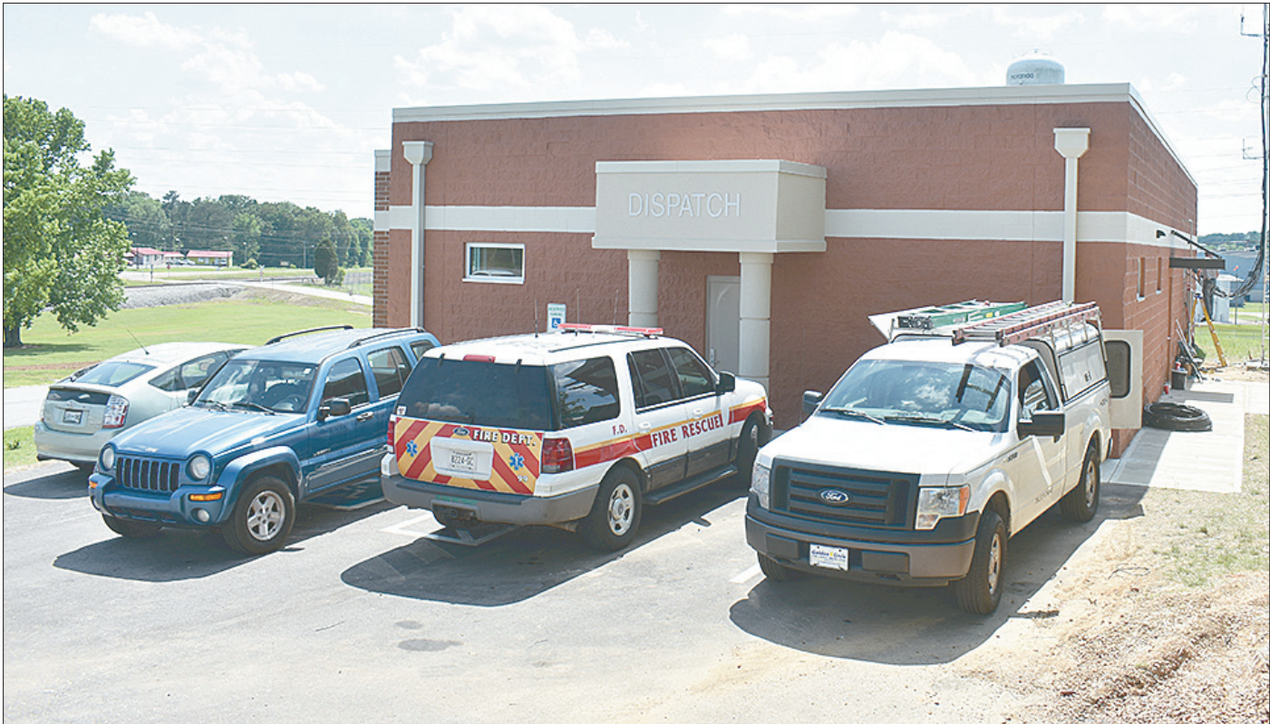
The Carroll County Emergency Operations Center houses the Emergency Management Agency, the Carroll County Fire Department and now the emergency services dispatch center, which is currently transitioning from its former location. Photo by Brad Sam/The Banner
