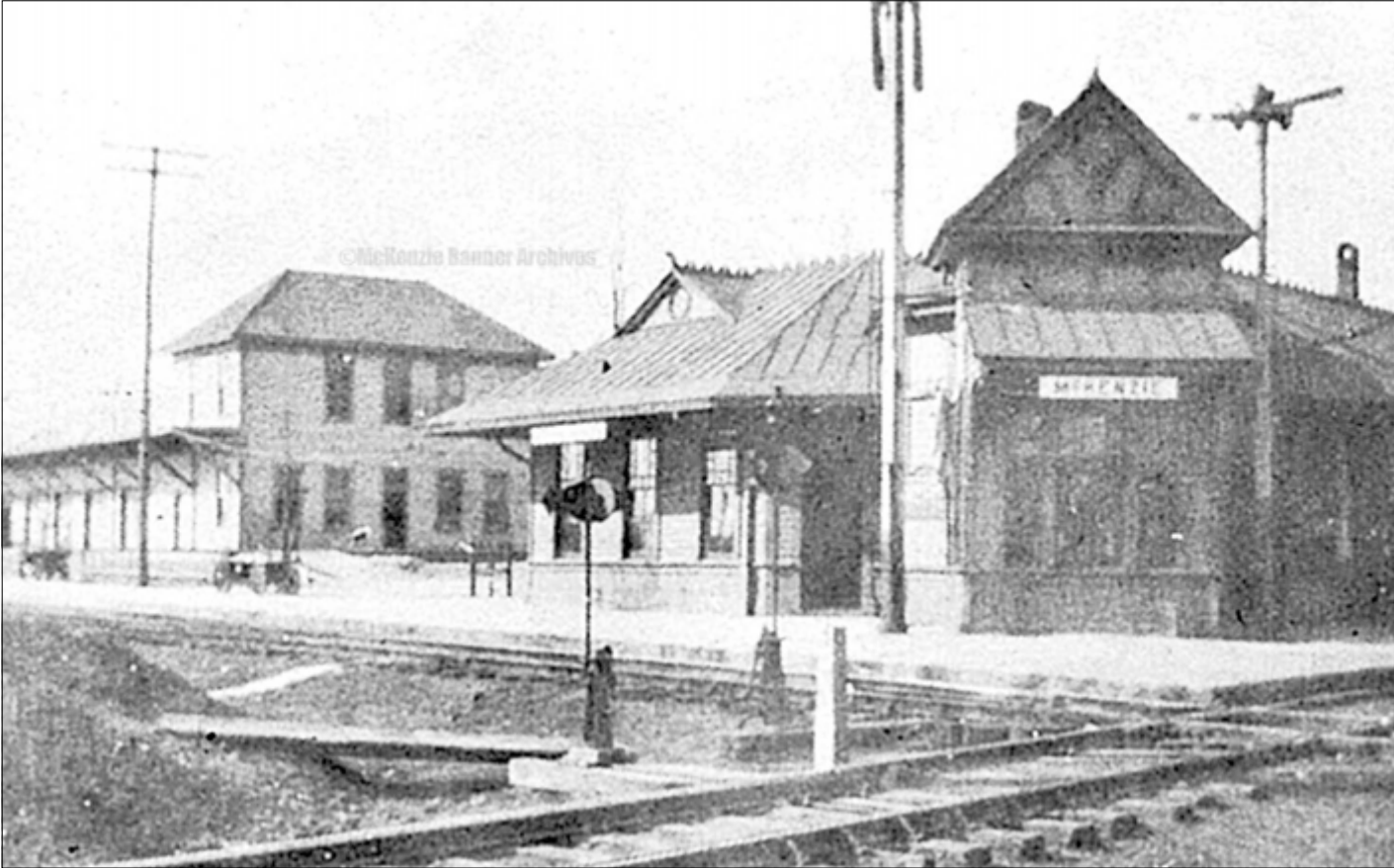
McKenzie Train Depot and Freight Loading Station in the early 1900s. File photo originally published in "A Pictorial History of McKenzie, Tennessee," by The McKenzie Banner in October 2004.
