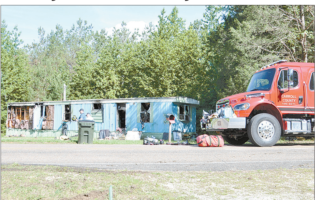
CARROLL COUNTY (June 1) — The Carroll County Fire Department extinguished a home fire Monday afternoon on rural Smyrna Road, southeast of Huntingdon. The blaze resulted in a total loss, but, fortunately, no one was injured. Photo by Brad Sam/The Banner
