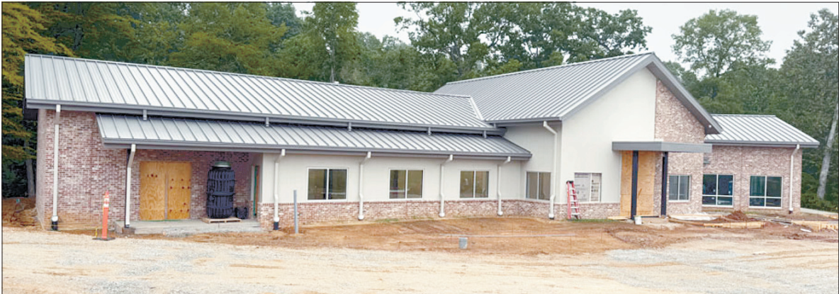
Construction on the new Carroll County 911 Headquarters in Huntingdon is still underway. Photo by Joel Washburn/The Banner
