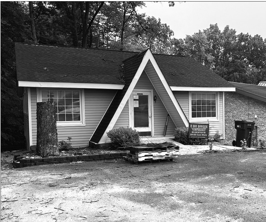
The former 911 administrative office (foreground) is to be razed to make way for the new headquarters on Dillahunt Lane, Huntingdon.
