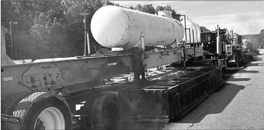
A massive convoy of road construction equipment works to 'mill and pave' State Route 22.
