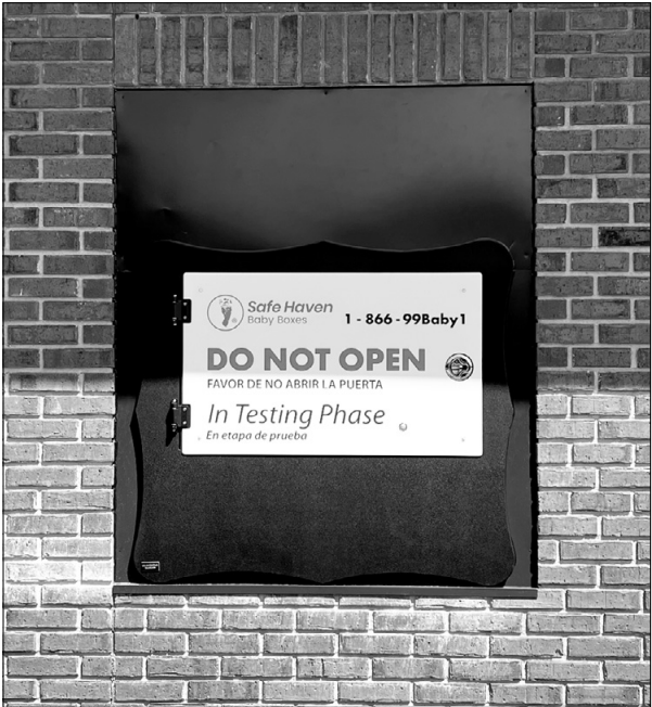
McKenzie's baby box is attached to the front-facing exterior wall of McKenzie's fire station. Photo by Lyndsey Summers/The Banner
