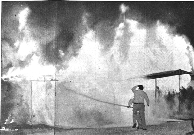
A grease fire early Monday evening at the Carroll Lake Country Club - virtually destroyed the two story frame building. The McKenzie Fire Department answered a call to the Country Club around 8 p.m. where a UT-Alumni meeting was being held. There were about 75 persons in the building who managed to escape unharmed. All the guests recovered their coats and purses before leaving the building only minutes before the structure was completely engulfed in flames. The fire originated in the kitchen while preparing steaks for the Alumni group. The grease caught on fire, spreading fire upward into the ceiling and rooftop area, according to the fireman's report. When the fire department arrived the entire building was completely out of control. Water from the swimming pool was used to quell the blaze. Some 45 minutes later firemen managed to contain the fire to the club area. Firemen managed to save a room that housed the swimming pool pump. Members of the Fire Department remained on the scene until 11:30 a.m.
