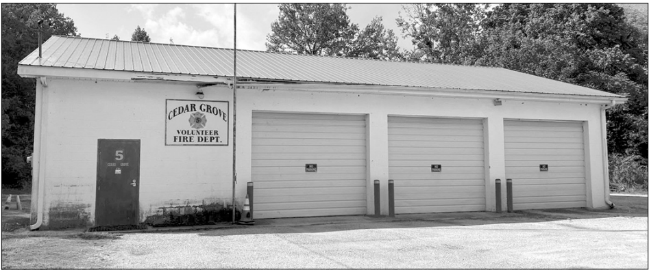
Cedar Grove Volunteer Fire Department.
