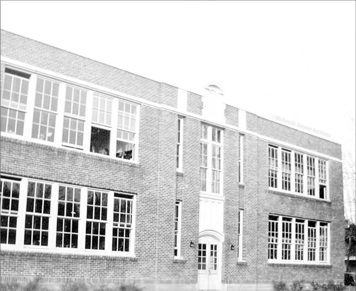
McKenzie Elementary School, Woodrow Ave., was constructed in 1937. File photo originally published in “A Pictorial History of McKenzie, Tennessee,” by The McKenzie Banner in October 2004.
