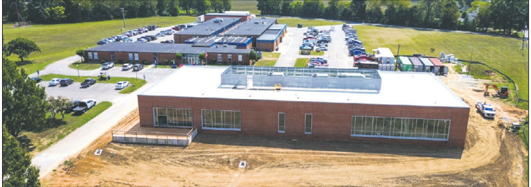
Aerial view of McKenzie's TCAT Henry/Carroll campus including the new facility still under construction. Photo from Bell Construction's Facebook page
