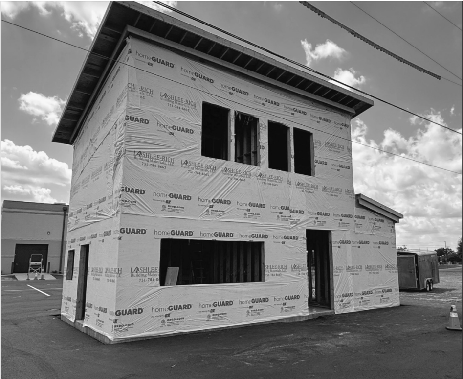
The new structure containing a concession stand, pressbox, restrooms, and ticket booth is under construction at the Mustangs’ baseball stadium.
