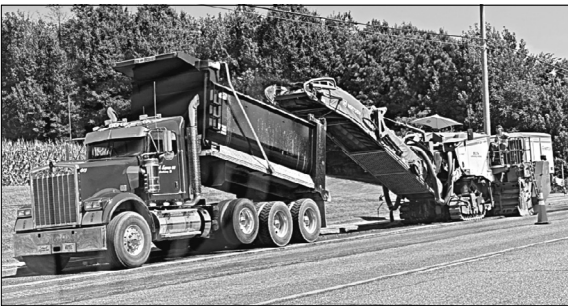
MCKENZIE — Construction crews began removal of the top layer of asphalt last week on U.S. 79 (S.R. 76) through McKenzie, ranging from the Henry County line then south just past Sydnor Road. Soon, paving crews will resurface the highway. Pictured is the pavement grinder removing the top surface.
