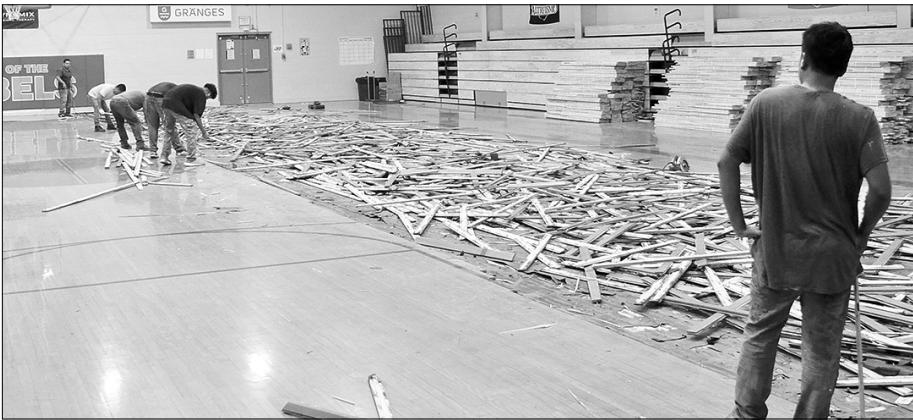
Workers with CQT Flooring remove the old flooring on Wednesday, July 16. Photo by Brad Sam/The Banner
