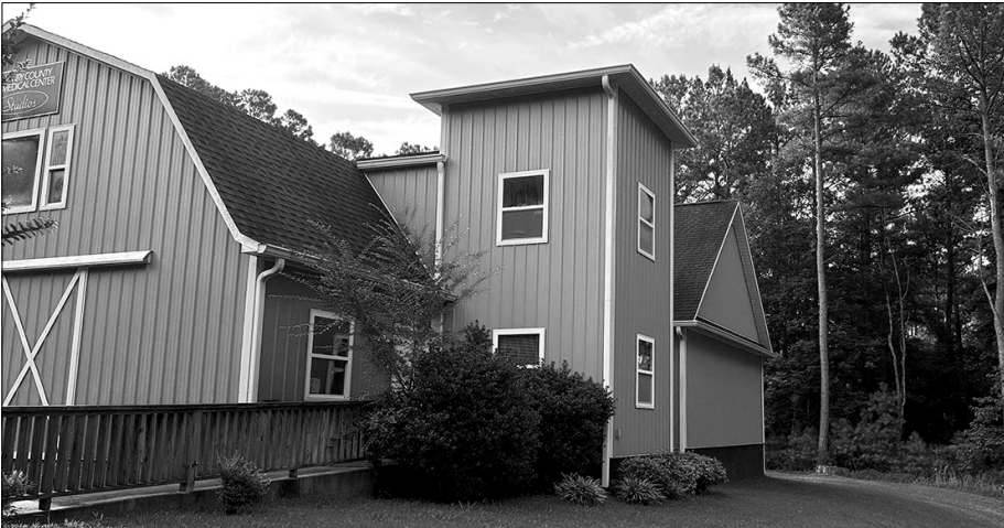
WEIO Studio located on Baker Road near Huntingdon.
