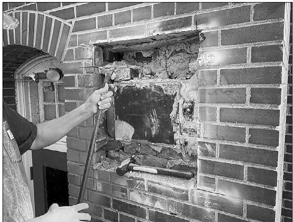
The copper cornerstone box found in the Dresden United Methodist Church was placed in 1923, and it could contain documents of Dresden's ancestry and religious history.
