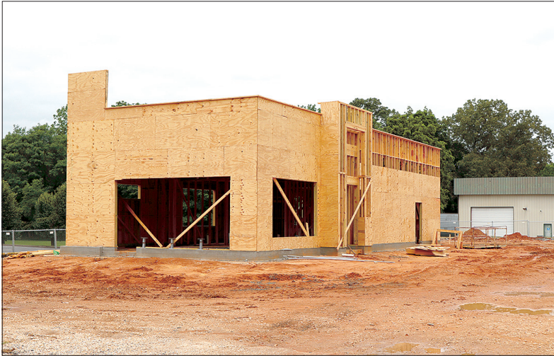
The basic frame of the new Taco Bell was in place on Memorial Day. Photo by Brittany Martin/The Banner
