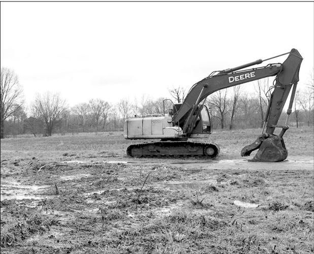
A trackhoe sits idle after razing a house along State Route 76 (US79) near Cutlip Lane in Trezevant. It was one of the many structures razed to clear a path for the new four-lane highway around Trezevant and Atwood.
