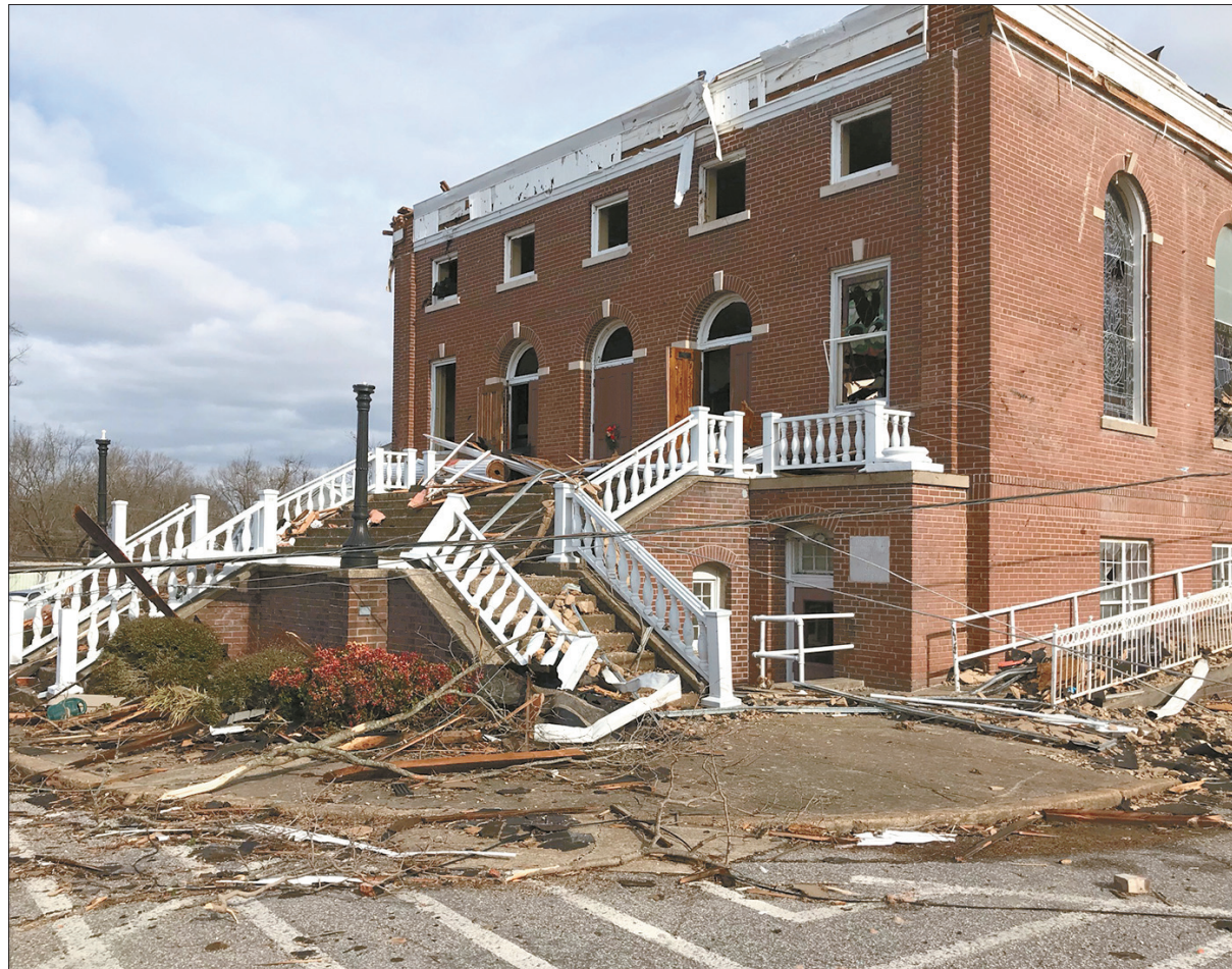
First United Methodist Church was heavily damaged in downtown Dresden. Photo by Brittany Martin/The Banner
