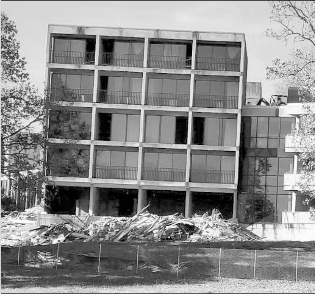
Workers are razing Paris Landing Inn to make way for a new inn scheduled to open in 2020. Photo by Shannon McFarlin
