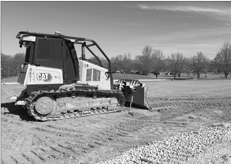
Earth-moving equipment is on site at the Highland Drive TCAT campus in McKenzie.
