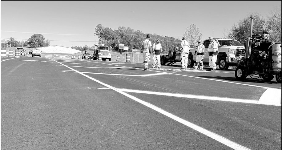
Construction crews add the final road markings on Monday morning prior to the official opening on Monday afternoon of the Atwood bypass road. Photo by Joel Washburn/The Banner
