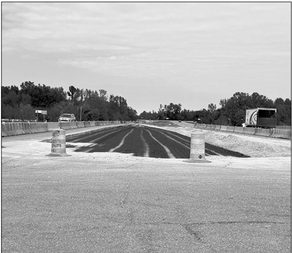
Highway 22 South-Huntingdon is undergoing an upgrade for turning lanes.
