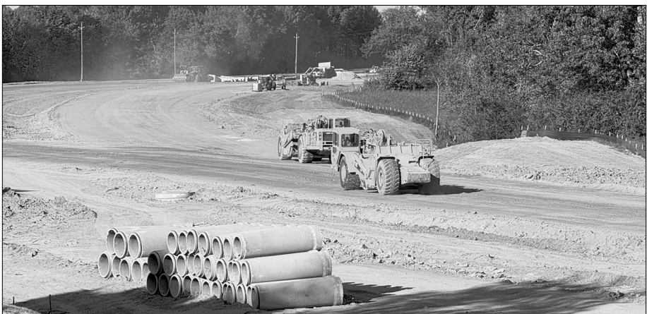
Earth-moving equipment is building the roadbed near Cutlip Lane just outside of Trezevant for the highway bypass that will bypass both Trezevant and Atwood.
